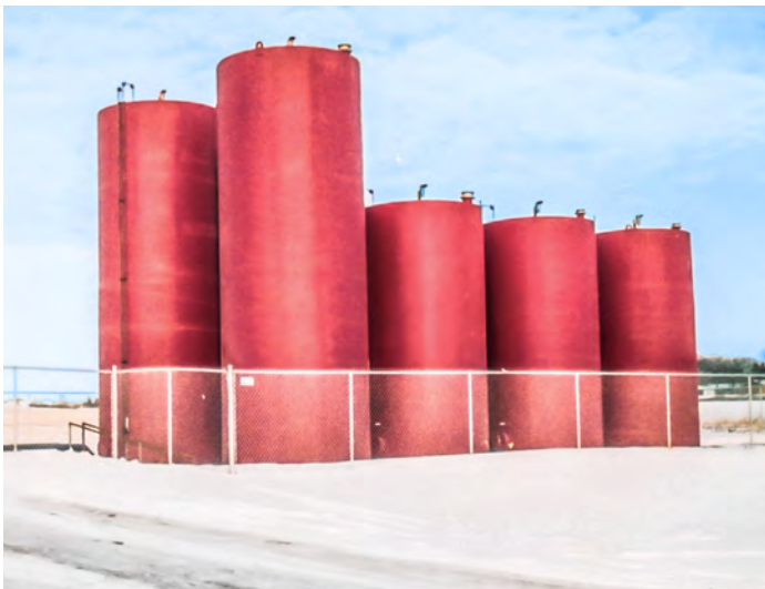
REFINED FUEL BULK PLANT
